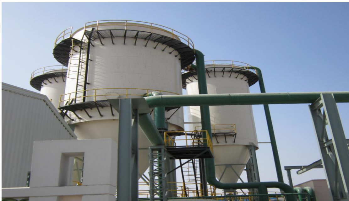
Fig. 6 Vertical settling tanks for sedimentation the marble slurry
